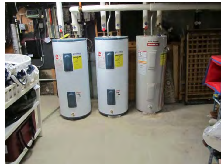
Each unit is equipped with its own electric domestic hot water tank located in the building's basement
