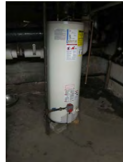
Freestanding natural gas-fired domestic hot water tank that serves the building's common areas
