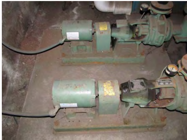
Base-mounted circulating pumps for distribution of hydronic heat
