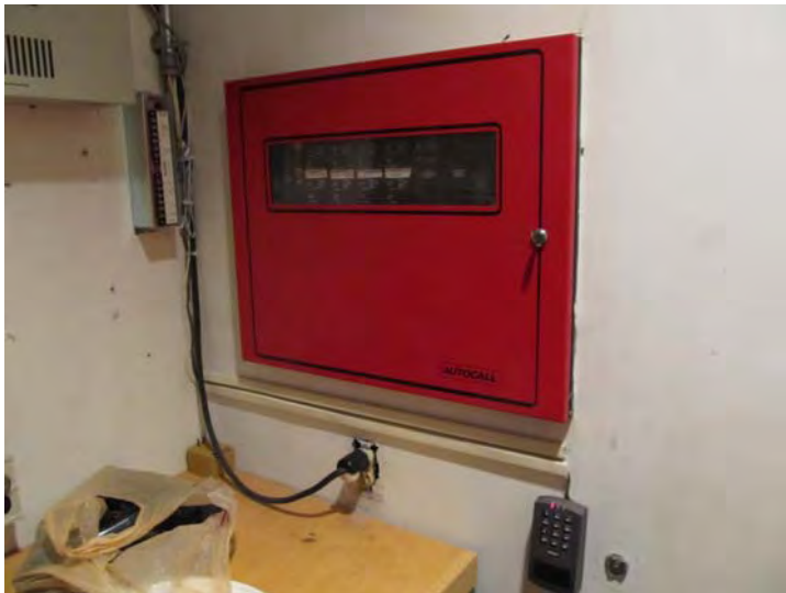
Zone-type fire alarm control panel – Equipment reportedly upgraded recently
