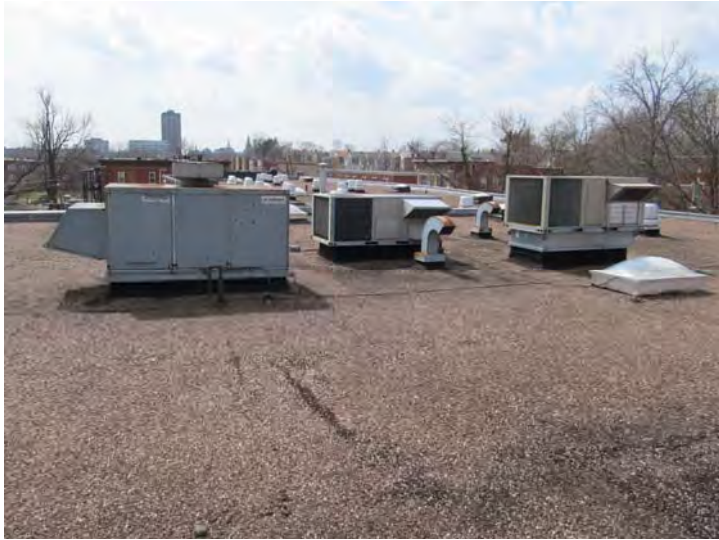
Rooftop-mounted make-up units providing heating and/or cooling for select interior common areas
