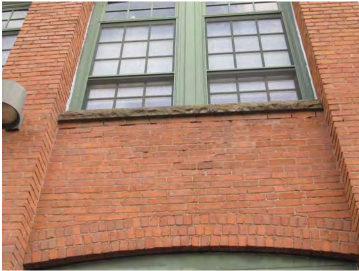
Loose and/or missing mortar noted under in brickwork at various locations around building
