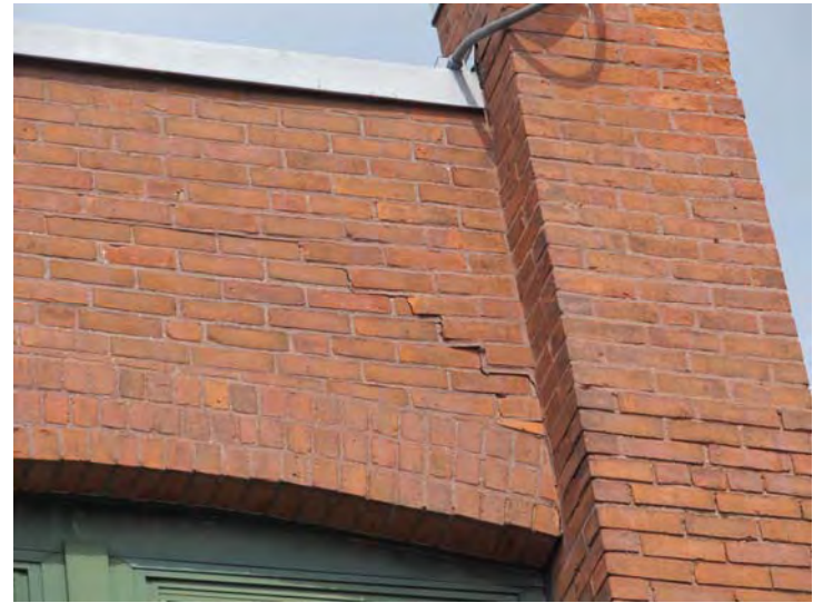
Isolated step cracks also noted at some locations
