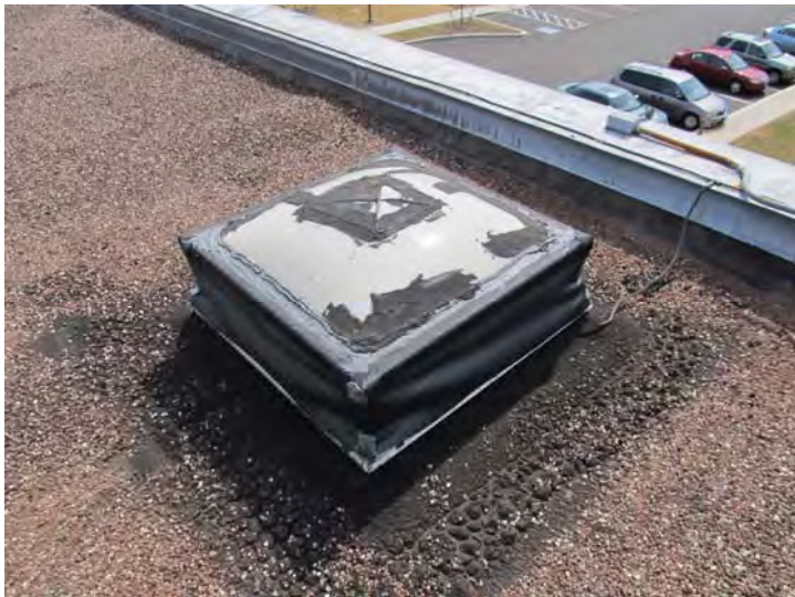
Skylights exhibit age-related wear and past repairs
