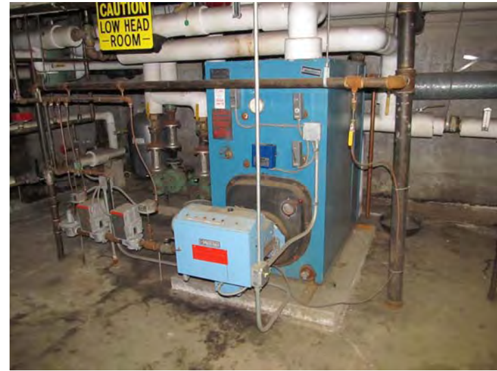
Original natural gas-fired boiler plant produces hydronic heat for the entire building
