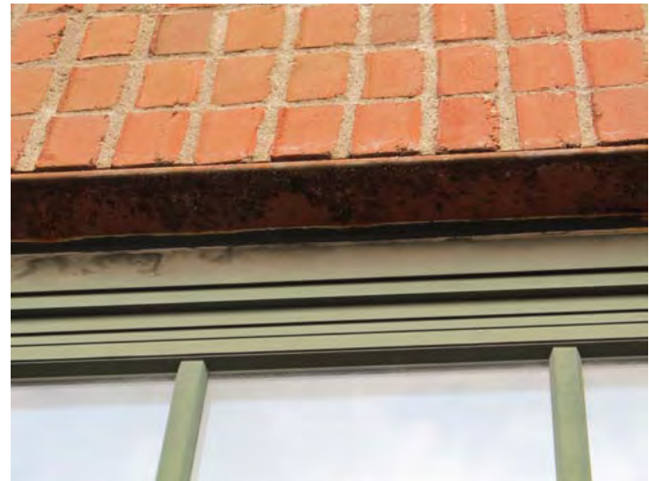
Steel lintels, present at some window openings, are in need of surface prep and painting
