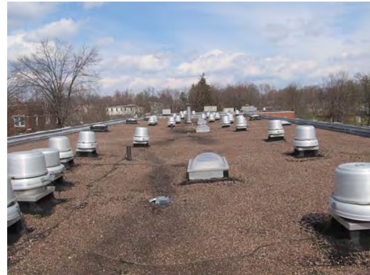
Built-up roofing system is nearing the end of its service life
